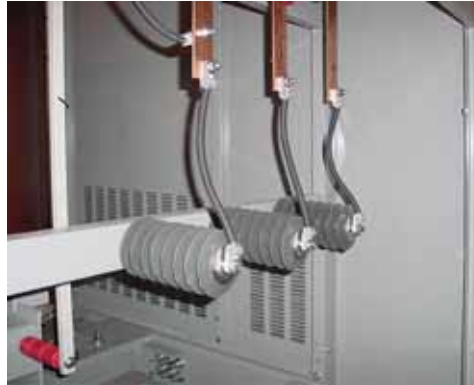
Figure 6: Installing Lightning Arresters
